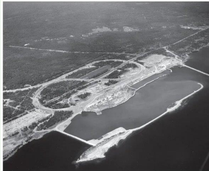
Aerial view of construction showing temporary road to Gull Island for breakwater construction.
