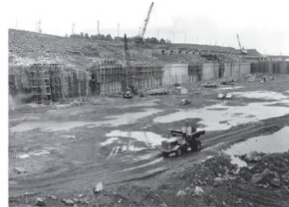
Constructing the dock face within the cofferdam thirty feet below the lake level.
