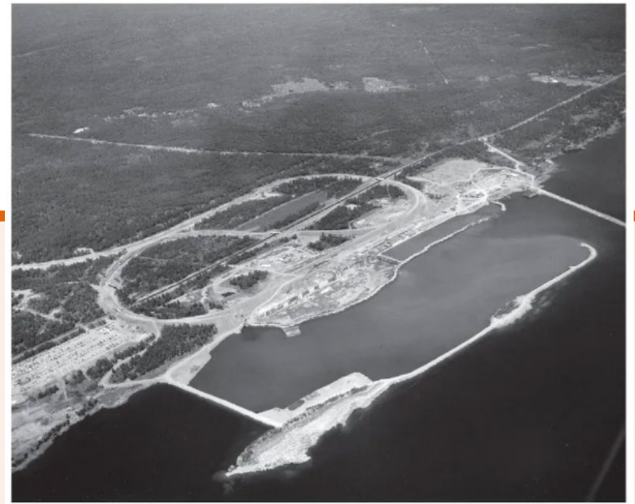
Aerial view of construction showing temporary road to Gull Island for breakwater construction.
